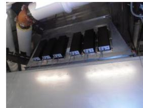
One advantage to the way the bi-polar ion technology is applied is that it requires no re-engineering of the HVAC system, requires no continual adjustment or maintenance except a replacement of the bi-polar ion tube every 2 years.
